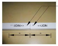
Finished Channel. The joined channels should now look like the picture with the CSJ positioned equally inside of the joined channels. Drill out holes with 3mm drill bit in CSJ to match the holes in channel and secure with the screws supplied. These may have to be temporarily removed during assembly.
