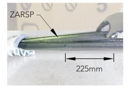
Step 2. Use the ZARSP to connect at the centre of the two ridge beams. Be sure it is pushed in fully.
